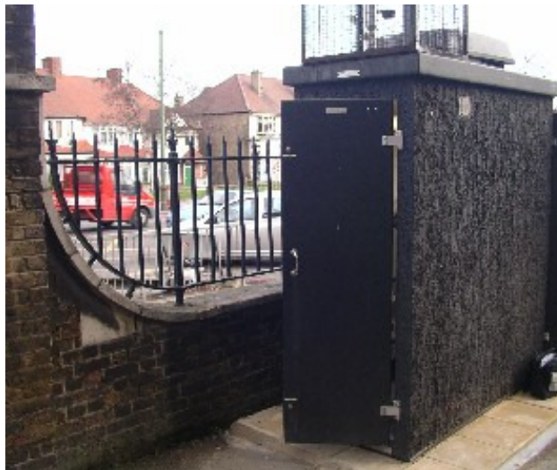
Figure 6 Enfield 5 monitoring site at Bowes Primary School (showing A406 in background)
